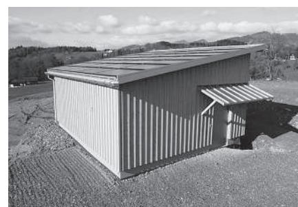
Photovoltaikanlage Reservoir Rüti
